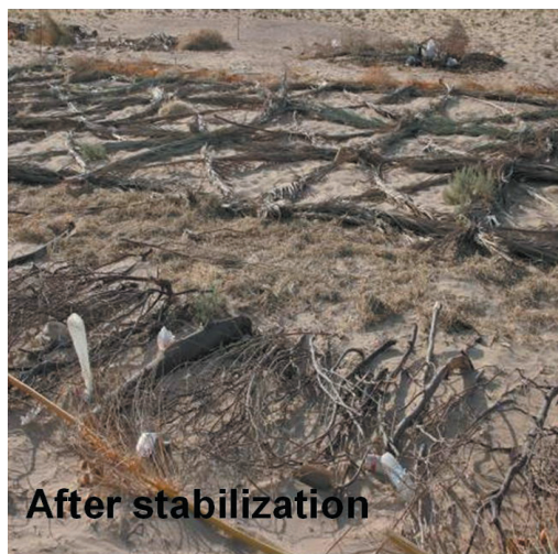
Figure 7. Soil Stabilization using environmentally friendly materials (Case of al Liyah)
