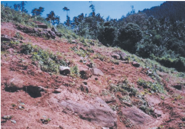
Figure 4. Eroded Land in the uplands
