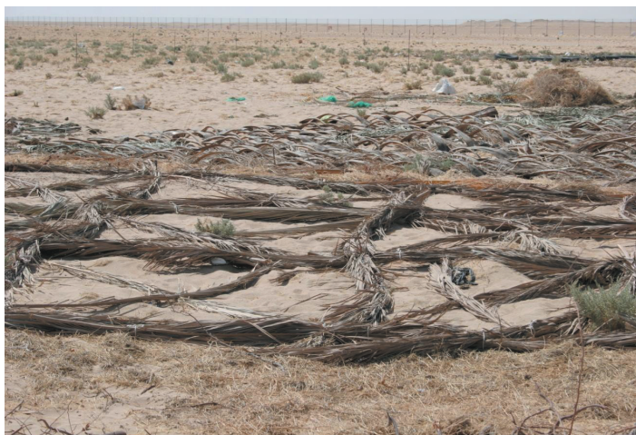
Figure 8. Using different parts of palm leaves in sand stabilization at Al-Liyah area, August 2006
