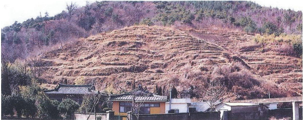
Before preventive erosion control
