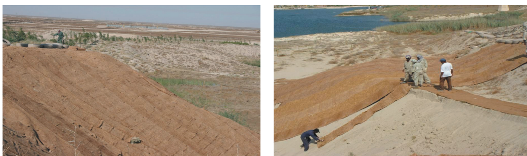
Figure 5 and 6. Using ecomat in stabilization of mobile sand body at KOC (Arabian Scientific Consultancy Center, Kuwait) November, 2006.
