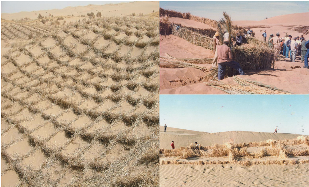
Figure 9. Application of plant residues (mainly palm leaves) in different designs to control shifting sands in arid regions
