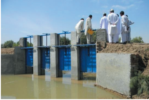
Figure 2 and 3. Gated structure along the main channel & Inlet structure on farm
