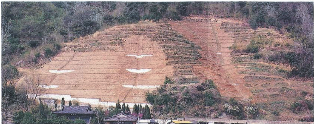
After preventive erosion control
