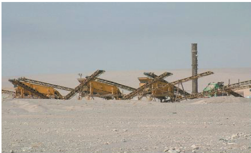
Figure 13. Refilling of gravel quarries at Liyah site
