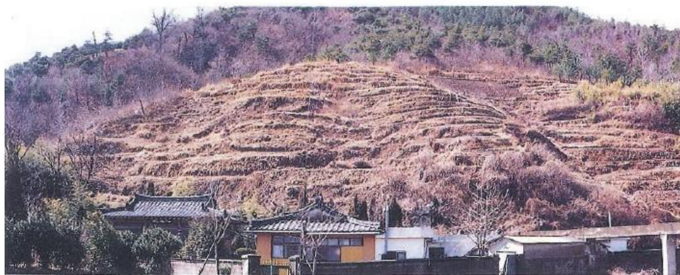
Before preventive erosion control
